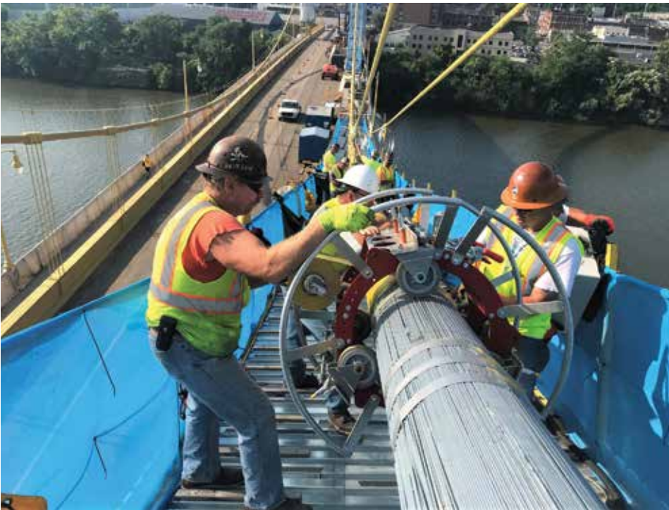
Workers on The Philip Murray Bridge. Credit Allegheny County.
