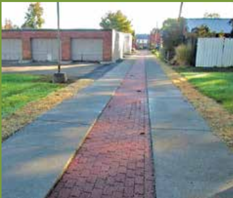
Limekiln Alley after.
