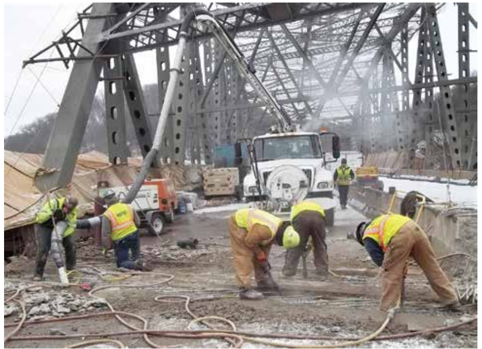
The Fleming Park Bridge receives work. Credit Allegheny County.
