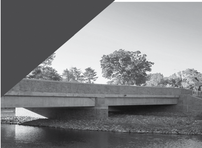
Experienced County Bridge Engineer
