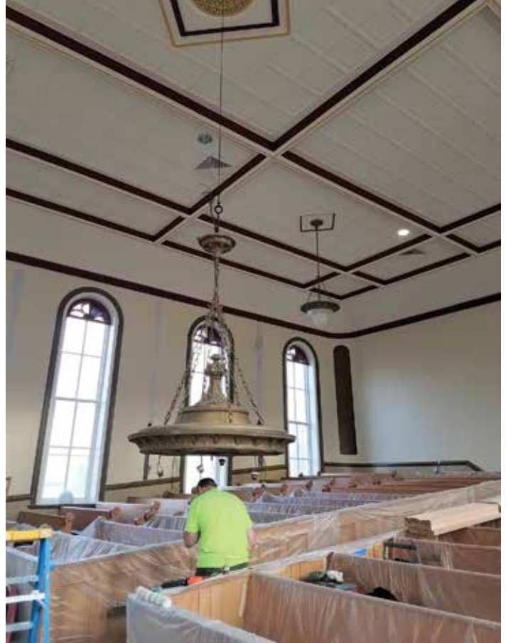
Clinton County courtroom chandeliers were brought down for rewiring and cleaning
