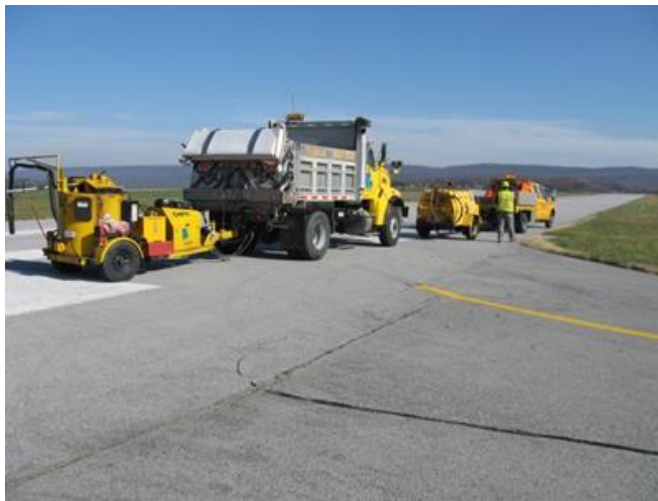
PennDOT provided crack sealing and line painting a County Airport
